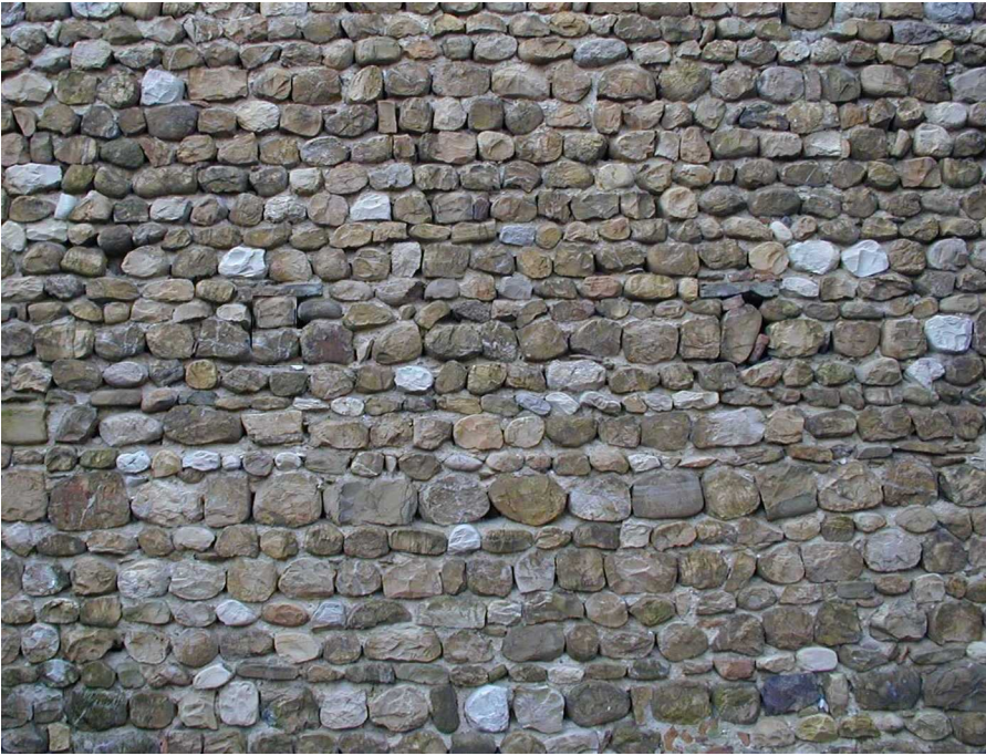
Figure 1. Portion of the medieval defense walls of an Italian town. Note that the hypothesis of periodic continuum is not applicable.
