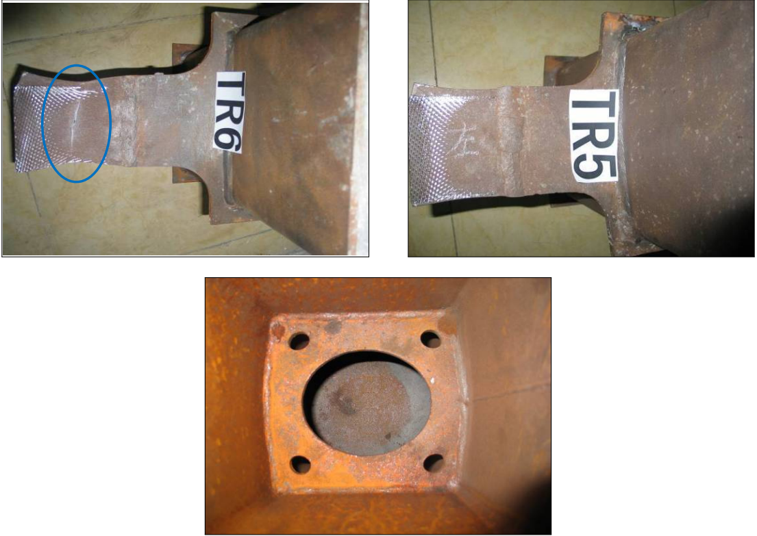
Figure 7. Failure modes. Clockwise from top left: fracture at steel beam flange; local buckling at steel tube; stretching of diaphragm.
