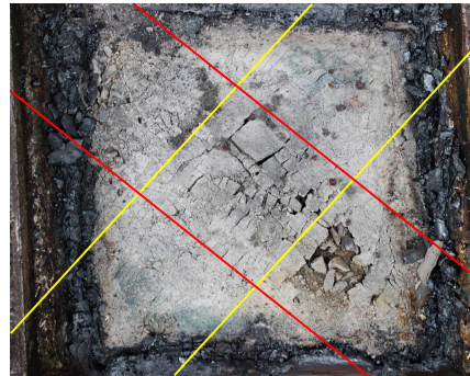
Concrete compression strut crushed
