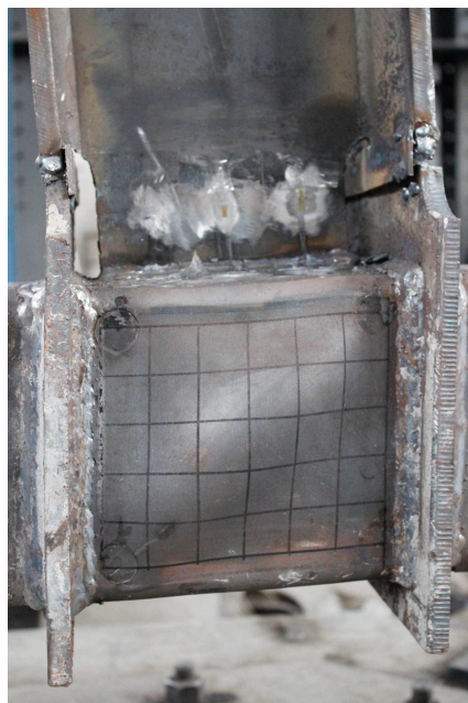
Bulged outward of column web
