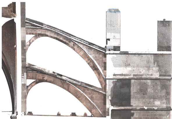
Figure 16. Orthophoto of south flying buttresses B1 (based on the cloud of points by Rex Haberland).
