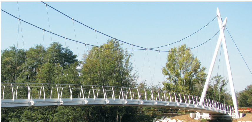
Figure 2. View of the Seriate footbridge.
