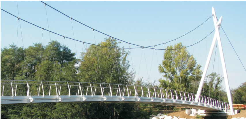
Figure 2. View of the Seriate footbridge.
