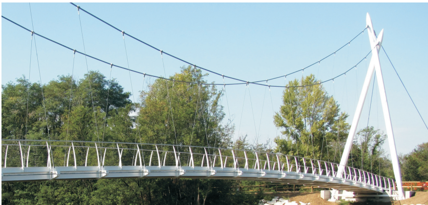
Figure 2. View of the Seriate footbridge.
