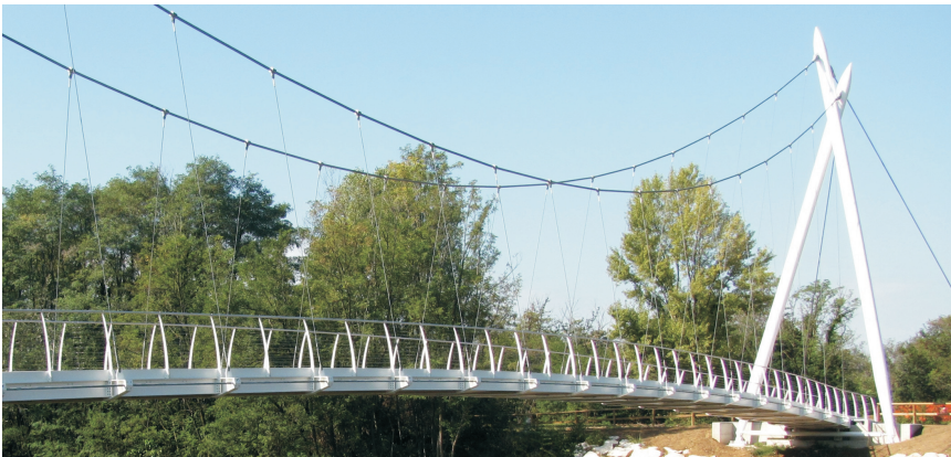
Figure 2. View of the Seriate footbridge.
