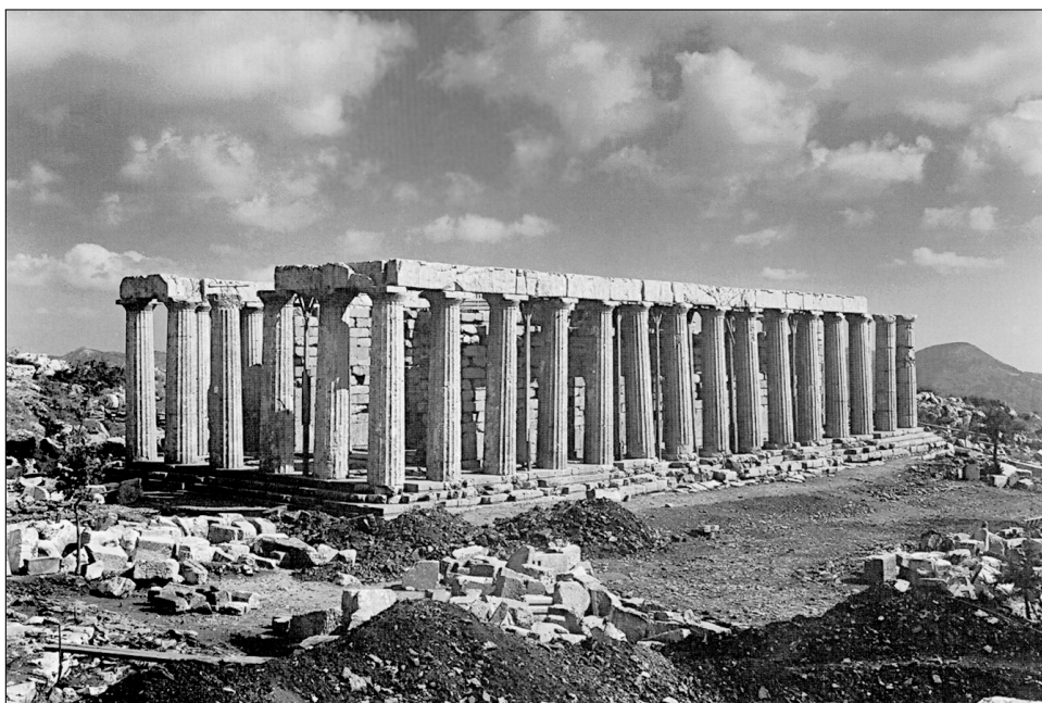
Figure 1. View of the temple of Apollo at Bassae from the north-west, before restoration work (Archive of the Ephoria Z, Olympia).
