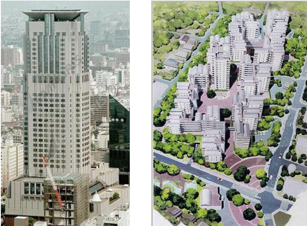
Figure 3. Left: Applause Building in Osaka, with a hybrid control system moving an heliport structure at the top. Right: sketch of the complex of 21 six- to fourteen-storey buildings erected on a unique “artificial ground” isolated at Sagamihara (Tokyo area) with 48 lead rubber bearings (LRBs), 103 sliding devices (SDs) and 83 ball bearings.
