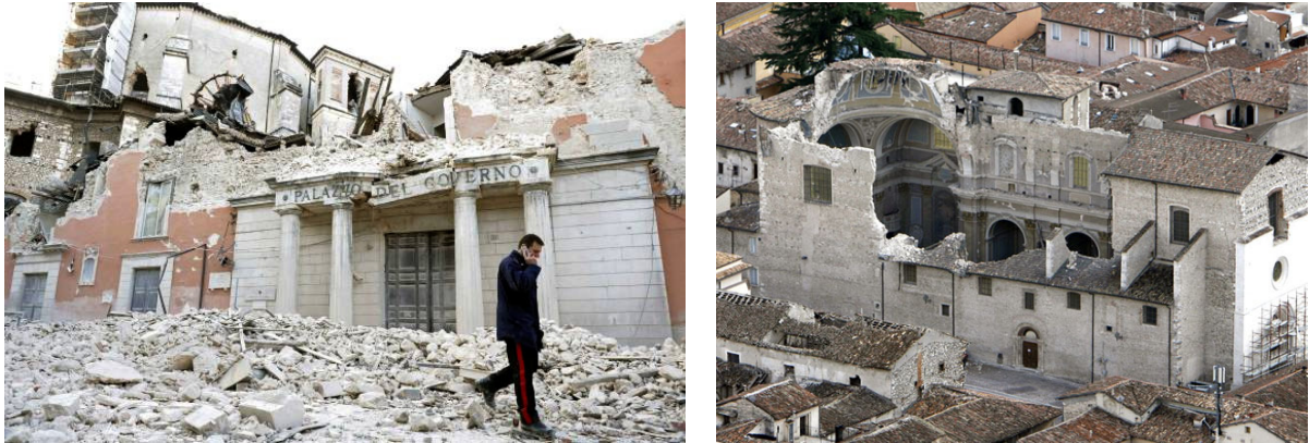
Figure 27. L'Aquila (April 2009): collapse of the Prefettura building (provincial headquarters of the national government) and the Santa Maria Paganica Church (right).
