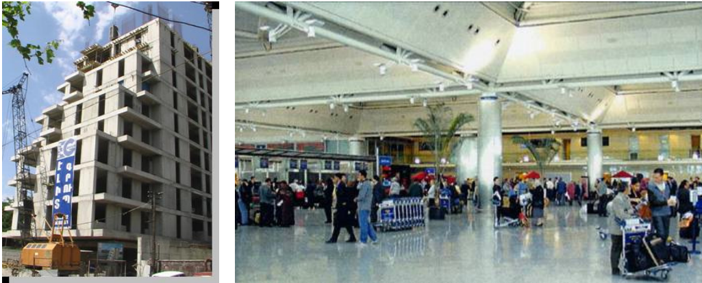
Figure 54. Left: the 15-storey Cascade multifunctional complex, isolated in Yerevan by MDRBs in 2006. Construction of even taller buildings is in progress. Right: the roof of the new Ataturk Airport in Istanbul, isolated by means of 100 FPS devices in 1999.
