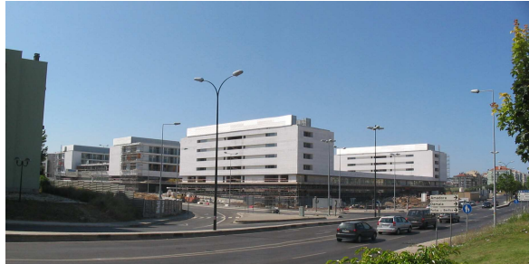
Figure 61. The new La Luz new hospital in Lisbon, which was base-isolated in 2006, together with a residence for old people, by means of 315 Italian HDRBs.
