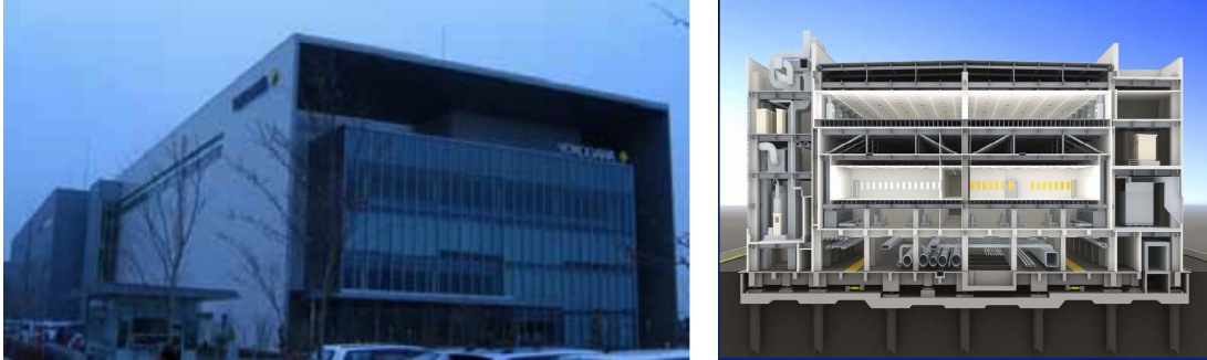
Figure 10. First seismically isolated Japanese factory for the production of semiconductors (height = 24.23 m, total area \approx 27,000 \text{ m}^2 ).
