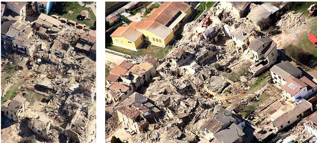
Figure 26. L'Aquila (April 2009): aerial views of some parts of the town where buildings collapsed or were heavily damaged.
