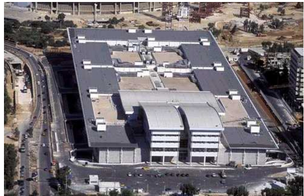
Figure 58. Left: the Rion–Antirion bridge in Greece, 12 km in length and protected, together with its approaches, by Italian SVPC devices, including 188 VDs. Right: the International Broadcasting Centre in Athens, isolated in 2003 by means of 292 Italian HDRBs.
