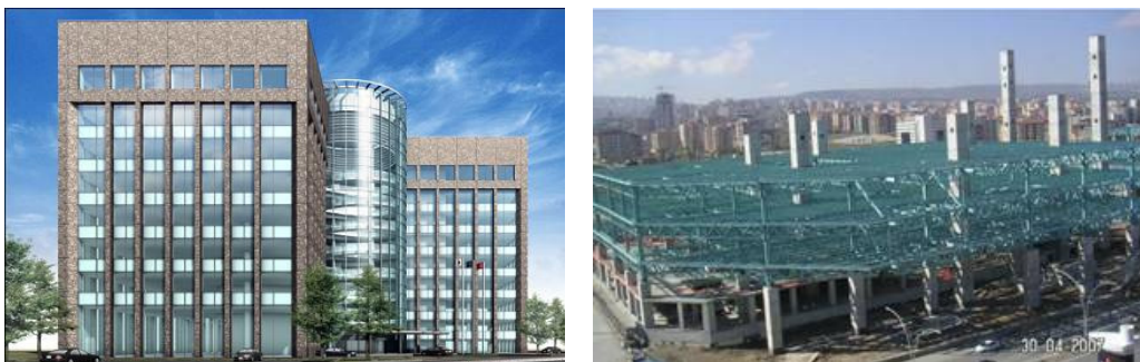
Figure 55. Isolated buildings in Turkey. Left: the T.E.B. Headquarters, a building which was under construction on 87 LRBs and LDRBs in Istanbul in 2006. Right: Söğütözü Congress and Commercial Centre in Ankara, isolated using 105 SIP devices manufactured in Germany in 2007.
