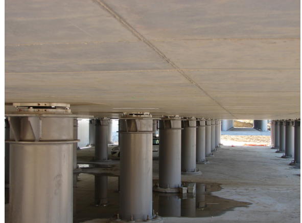
Figure 44. One of the 184 seismically isolated pre-fabricated houses erected at L'Aquila for homeless residents and CSS devices installed to isolate its supporting slab.
