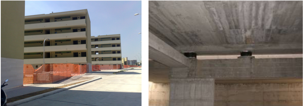
Figure 42. The four r.c. residential buildings of the new San Samuele Quarter of Cerignola (Foggia), in seismic zone 2, first application of the new Italian seismic code to isolated dwelling buildings, completed with 124 HDRBs (right) in May 2009, with safety certification of A. Martelli.
