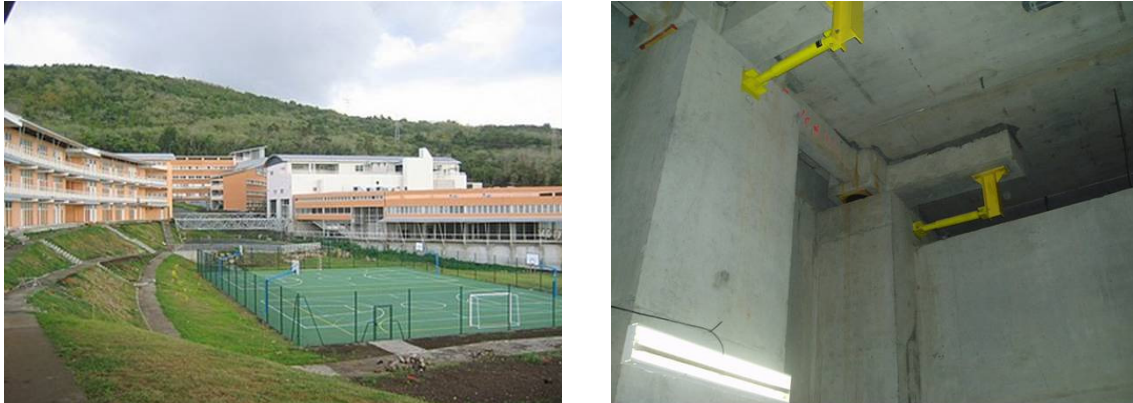
Figure 50. An isolated school in the French Martinique island (France), with a view of some NBs and VDs that protect it.
