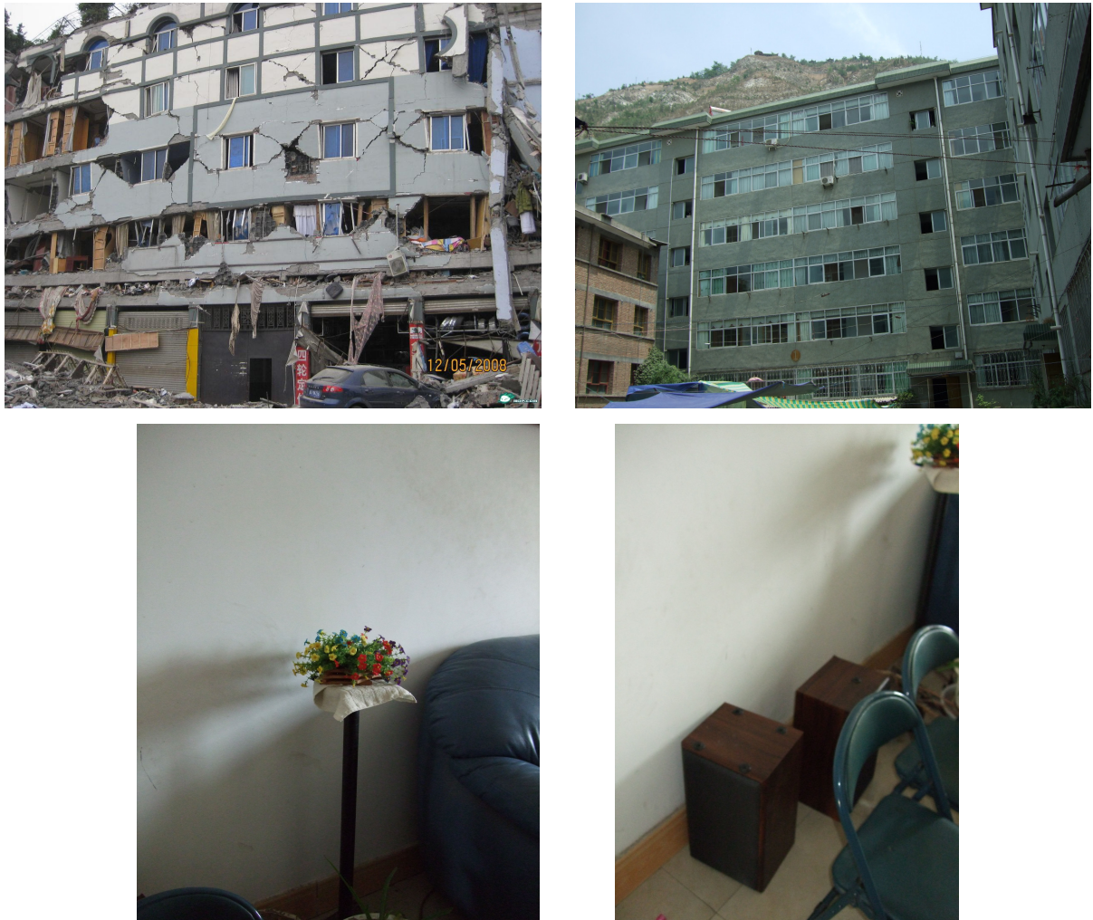
Figure 14. Top left: heavy damage was inflicted on this conventionally founded r.c. building by the 2008 Wenchuan earthquake; the building had been designed to withstand events of intensity I_{MMS} = 7 . Top right and bottom: this isolated building remained free of structural and nonstructural external and internal damage after the same earthquake.
