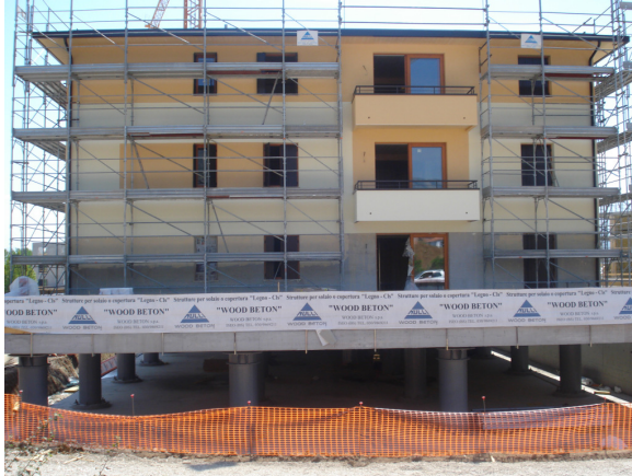
Figure 44. One of the 184 seismically isolated pre-fabricated houses erected at L'Aquila for homeless residents and CSS devices installed to isolate its supporting slab.
