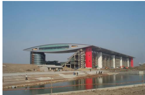
Figure 16. Left: Chinese stadium (23,000 m 2 ) protected by RBs and VDs, for which SI reduced the seismic response by a factor of 4.2. Right: and roof SI of the News Centre and Restaurant of Shanghai F1 Autodrome.
