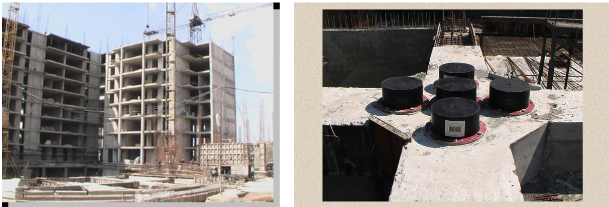
Figure 53. Left: the Our Yard multi-functional complex in Yerevan, with 10 to 16 storeys, was isolated in 2006 by means of MDRBs. Right: a group of such bearings.
