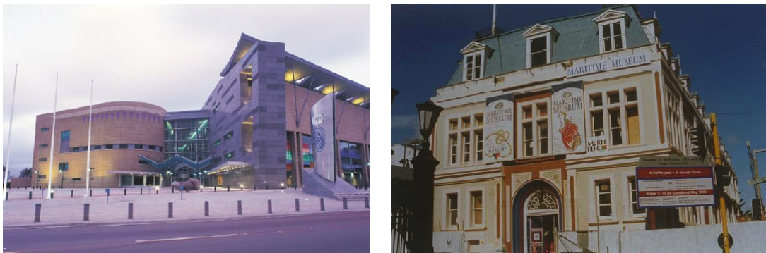
Figure 52. Wellington, New Zealand: the isolated Te Papa Museum (left) and the Maritime Museum (right), retrofitted with SI in 1993.
