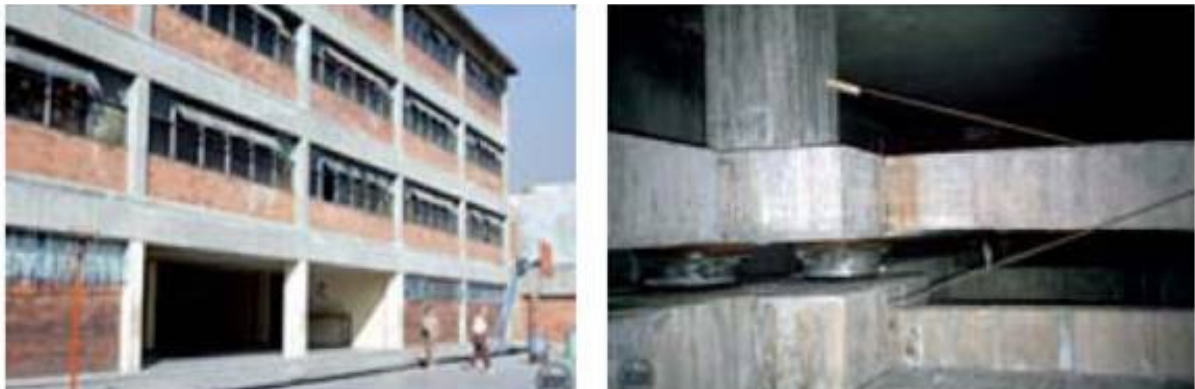
Figure 56. The Legaria Secondary school at Mexico City (first Mexican application of SI, performed in 1974) and one of its rolling SI devices, developed in Mexico.
