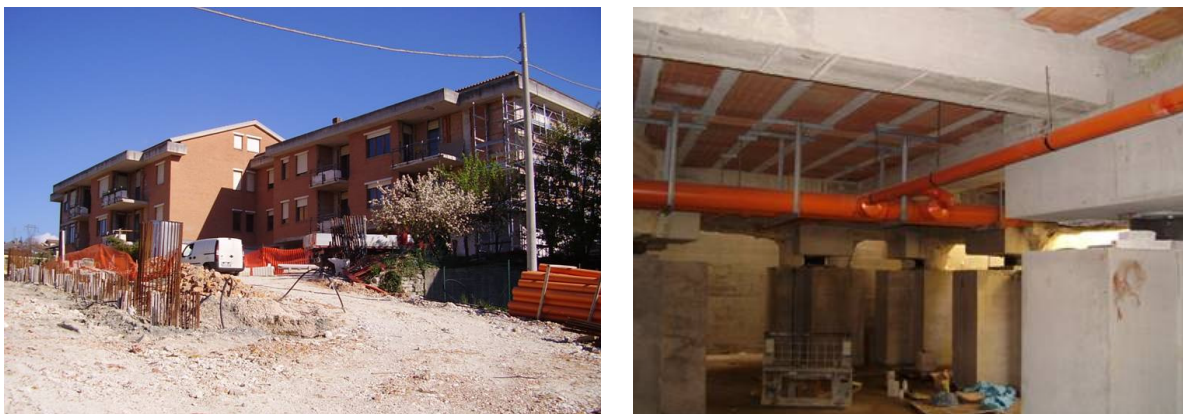
Figure 33. Three-storey r.c. private house in Fabriano (Ancona), in seismic zone 2, damaged by the 1997–98 Marche and Umbria earthquake. It is the first EU application of SI in a subfoundation, the retrofit of which was completed with 56 HDRBs of three sizes in 2006, with safety certification by A. Martelli.
