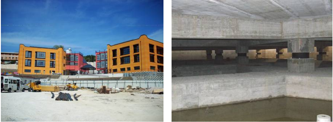
Figure 36. The new Francesco Jovine primary school and Le Tre Torri Professional and University Centre, erected in San Giuliano di Puglia (seismic zone 2 since 2003) on a single seismically isolated slab, and its SI system (61 HDRBs and 12 SDs) during construction. The isolators were donated by the Italian ALGA, FIP Industriale and TIS manufacturing companies. The SI design is by a team of experts coordinated by the GLIS and ASSISi member P. Clemente of ENEA, with tests done by the University of Basilicata. Safety was certified by A. Martelli and GLIS member C. Pasquale in September 2008.
