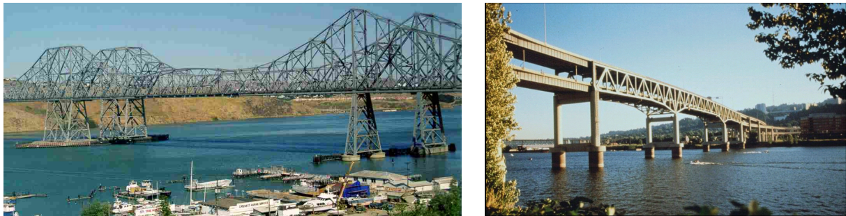
Figure 18. Left: Carquinez Bridge, California, retrofitted by means of Italian STUs. Right: Marquam Bridge, Oregon, retrofitted by means of Italian RBs and EPDs.
