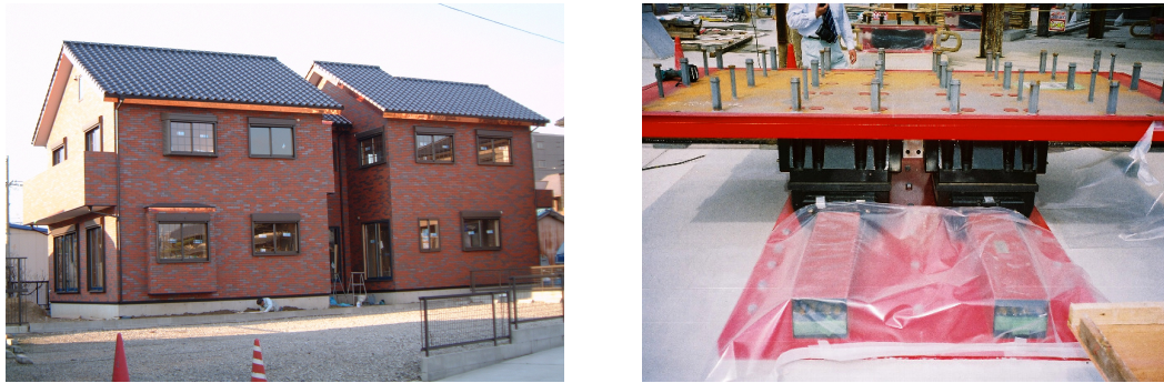
Figure 6. A Japanese private house protected by an SI system formed by steel sphere recirculation isolators, viscous dampers (VDs) and recentering devices.
