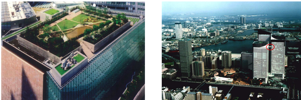
Figure 7. Left: “green mass damper”, used as the TMD of a 45 m tall building of the Keyaki-zaka residential complex, in Tokyo. The garden base is 1 m thick, weighs 3,650 t, or 8% of the building mass, and is supported by 46 rubber bearings (RBs) and 22 visco-elastic dampers (VEDs). Right: ADB between Japanese high-rise buildings.
