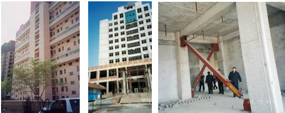
Figure 11. The tallest seismically isolated Chinese building (19 storeys), erected at Taiyuan City, in Northern China (left), and a Chinese high-rise building protected by VDs (center and right).
