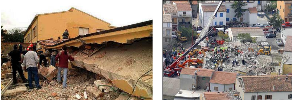
Figure 24. Collapse of the Francesco Jovine primary school in San Giuliano di Puglia (Campobasso) during the 2002 Molise and Puglia earthquake, and search for survivors amid the debris.
