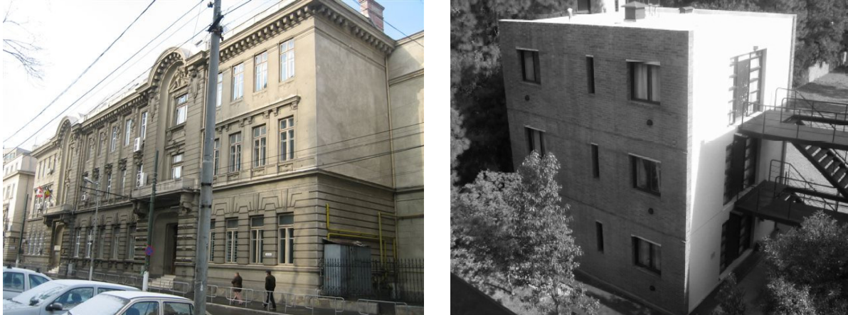
Figure 66. Left: retrofit design with SI of the Victor Slavescu monumental building in Bucharest, Romania, erected in 1905 (55.2 m \times 20.87 m; height = 22.5 m). Right: residential building for university students at Mendoza, Argentina, isolated by means of four 3D German GERB isolators.
