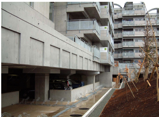
Figure 4. Lateral view of the isolated building complex of Figure 3 and the large garage located below the artificial ground plate, with the isolators protected from fire (the SI system lowers the period of the 111,600 t superstructure to T = 6.7 s, with a design displacement of 800 mm).
