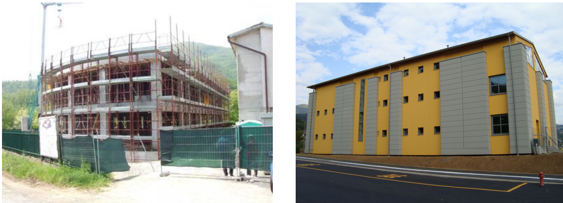
Figure 37. The first new school building of Mulazzo (Massa Carrara), protected by LRBs and SDs (right) and the new primary and secondary school of Galliciano (Lucca), protected by HDRBs and completed in September 2009. They are two of the 5 schools rebuilt or being rebuilt with SI in Tuscany, in seismic zones 2. Safety of the Mulazzo school will be certified by A. Martelli, that of the Galliciano was certified by A. Parducci.
