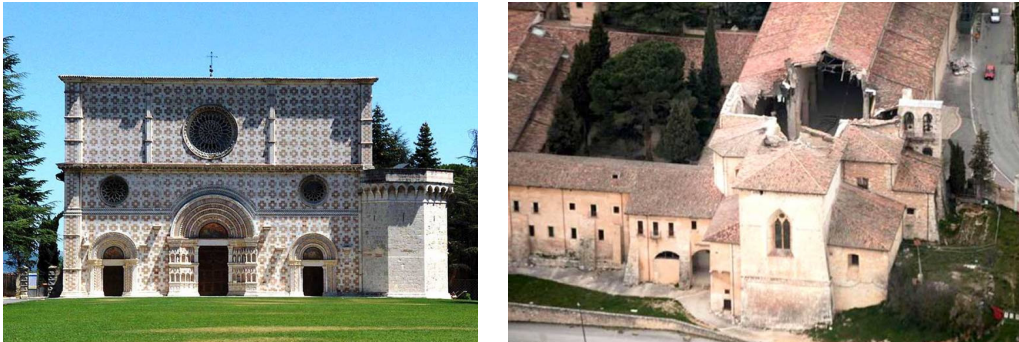
Figure 28. The Cathedral of Santa Maria di Collemaggio, a rare example of Abruzzo Romanesque style, prior to the earthquake, and the collapse of the roof of its baroque (not yet retrofitted) part. The façade, which had been protected by some EPDs installed on the roof some years earlier (see Figure 45), survived the earthquake; however, a steel scaffold, previously erected for an already planned retrofit, certainly helped.
