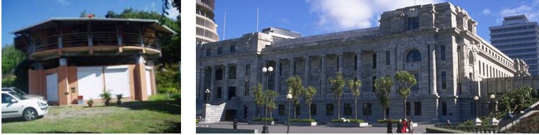
Figure 51. Left: a small seismically isolated building in the French Martinique. Right: the New Zealand Parliament at Wellington, a historic building erected in 1921 and retrofitted using LDRs in 1992–93.
