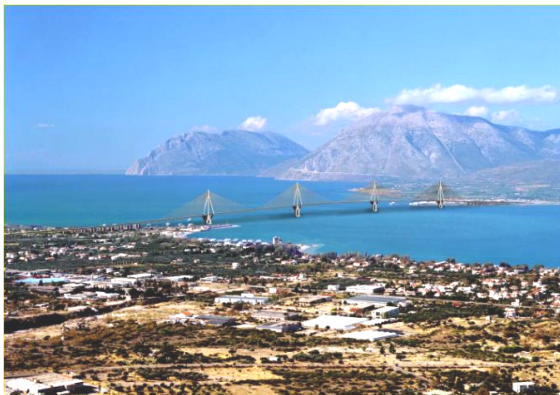
Figure 58. Left: the Rion–Antirion bridge in Greece, 12 km in length and protected, together with its approaches, by Italian SVPC devices, including 188 VDs. Right: the International Broadcasting Centre in Athens, isolated in 2003 by means of 292 Italian HDRBs.
