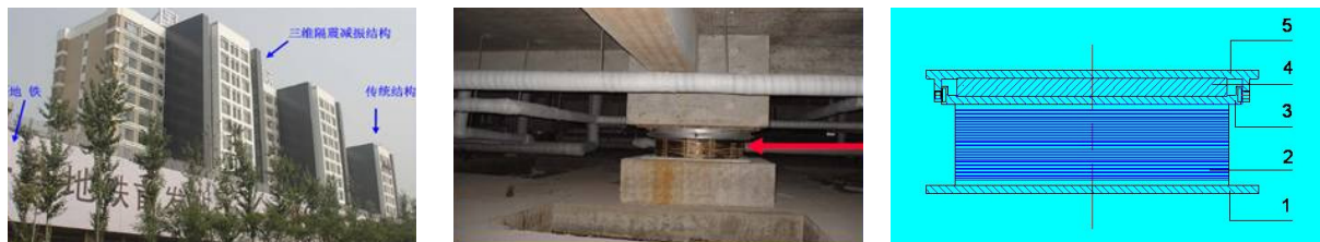
Figure 12. Left: new Chinese buildings protected at Guangzhou by 3D RBs from both horizontal seismic vibrations and vertical traffic vibrations. Center: one of the 3D RBs. Right: its sketch (4 = vertical element). Similar applications exist in Beijing.
