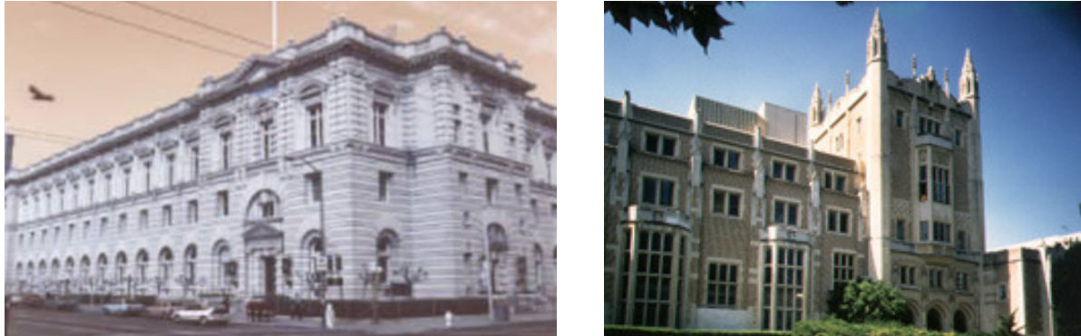
Figure 23. Further US building retrofits with SI. Left: San Francisco Court of Appeal, retrofitted with FPS. Right: Kerckhoff Hall at the University of California, Los Angeles (total living area = 8,300 m 2 , 6 storeys).
