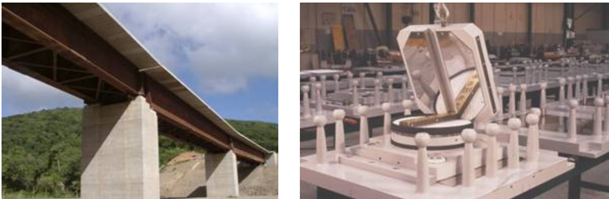
Figure 64. The Caracas – Tuy Medio railway in Venezuela (26 isostatic span viaducts, overall length = 7,775 m, 217 spans), protected by over 1,500 isolators manufactured in Italy in 1999–2003.
