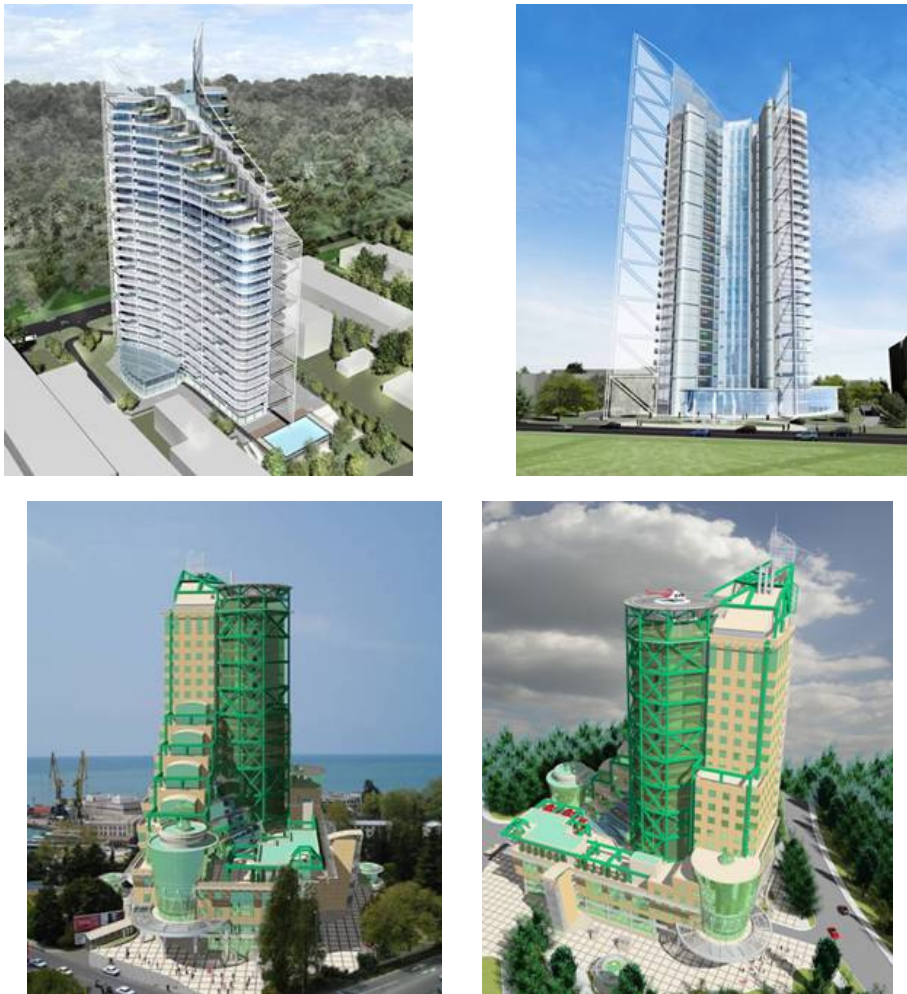
Figure 17. Top: new Sea Plaza Hotel at Sochi (27 storeys, in addition to 2 underground ones; height \approx 93 m; total living area = 40,000 \text{ m}^2 ), protected by 102 HDRBs. Bottom: new r.c. commercial center, with cinema, underground parking and offices, again at Sochi (21 storeys, in addition to the ground and 2 underground floors; height \approx 100 m; total living area = 50,000 \text{ m}^2 ), protected by 200 LRBs.
