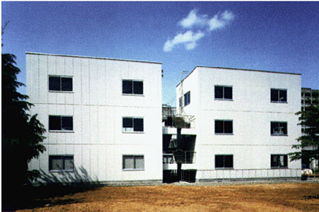
Figure 10. Test buildings at Tohoku University. Left: conventional seismically designed building; right: seismic isolated building.
