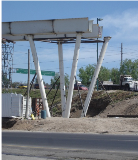
Figure 14. Bridge during construction.
