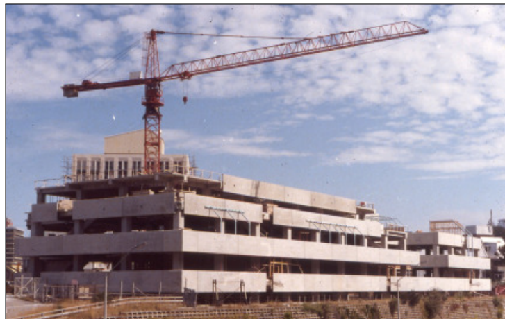
William Clayton Building under construction, 1981.
