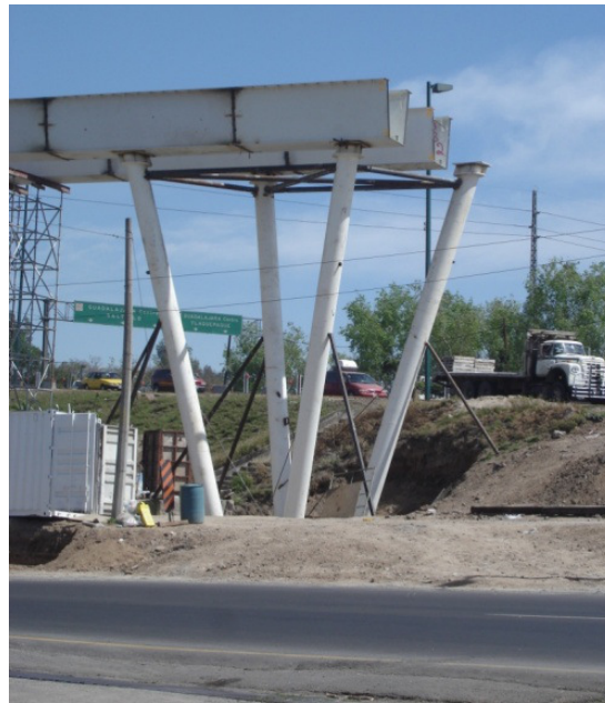
Figure 14. Bridge during construction.
