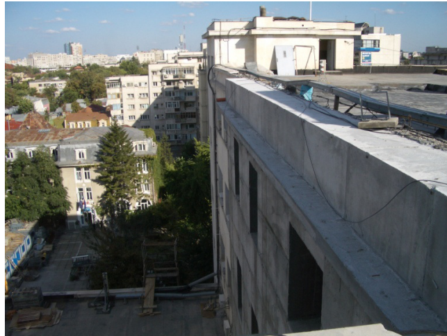
Figure 28. New shear wall.
