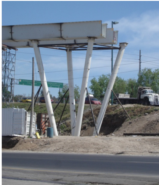
Figure 14. Bridge during construction.
