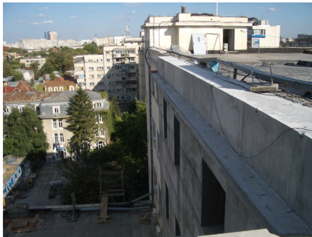
Figure 28. New shear wall.
