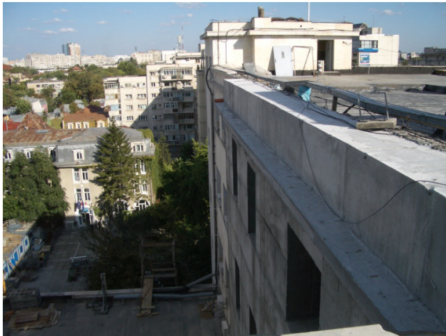
Figure 28. New shear wall.
