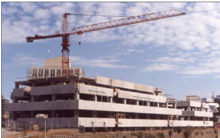
William Clayton Building under construction, 1981.
