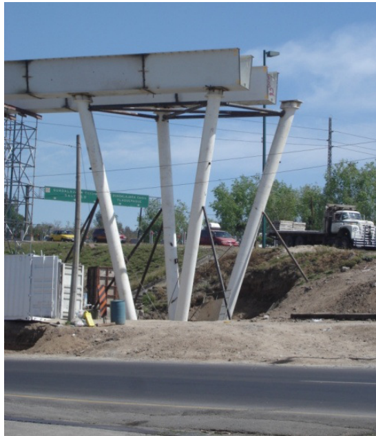
Figure 14. Bridge during construction.
